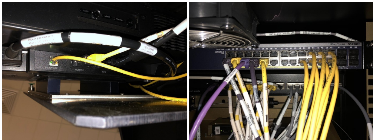
Figure 2-49. Connections from a Projector to the Display Switch
